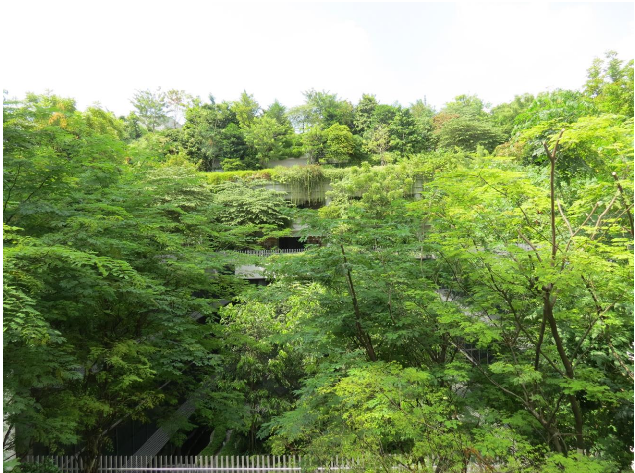
Figure 3. Part of the rooftop garden of the Kampung Admiralty development.
