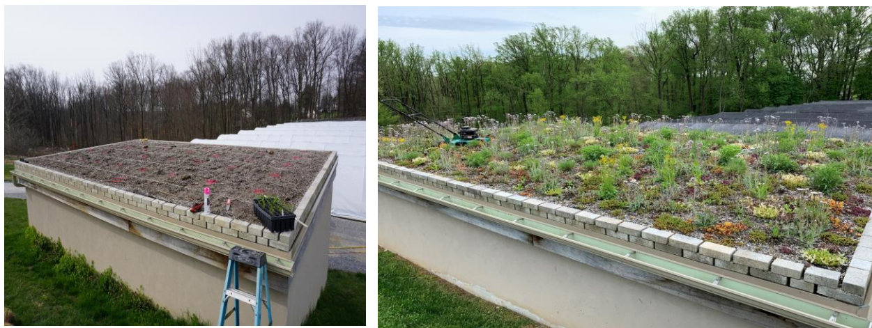
Figure 4. Establishing a green roof in Landenberg, Pennsylvania.
