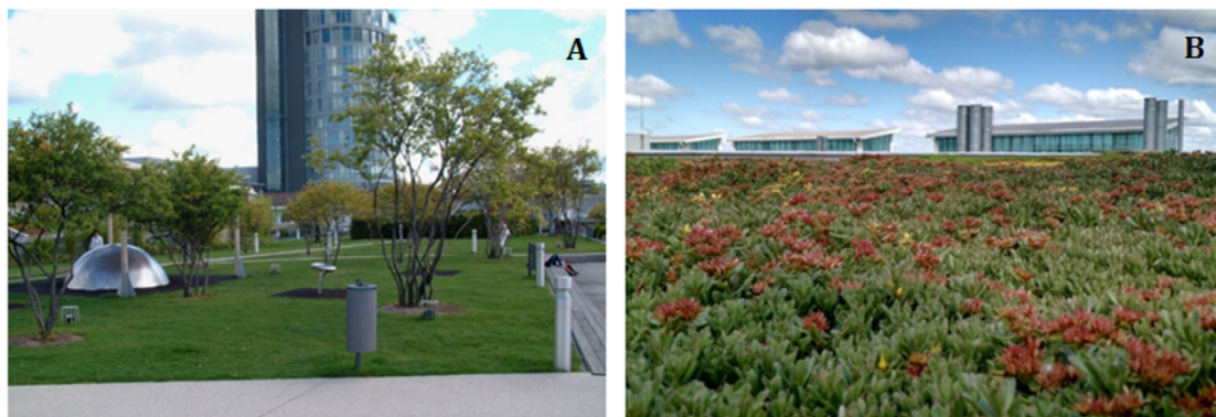
Figure 1. A: An intensive green roof at the Schlossle Galerie in Pforzheim, Germany. B: Portion of a 10.4 acre extensive green roof on a truck assembly plant at Ford Motor Company in Dearborn, Michigan.
