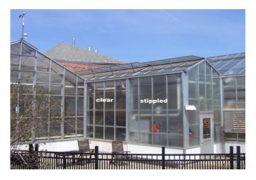
Figure 1. Clear and stippled greenhouse glass.
