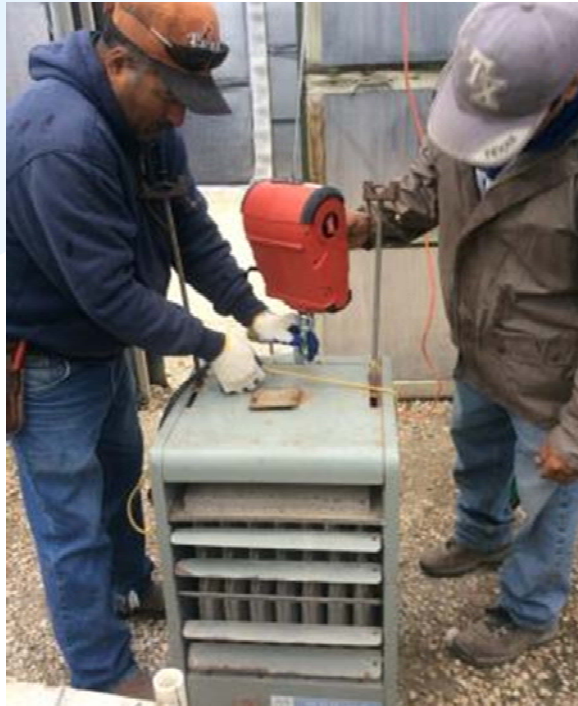
Hooking up Heater to Winch
