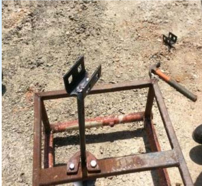
Anchor and Install Brace
