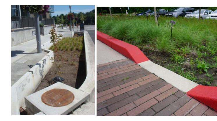
Figure 3. The idea is to "peel back" the city's concrete and asphalt and replace it with plants – via rain gardens, green roofs, heavily planted curb extensions, vegetated "swales" in parking lots, and mini-wetlands.
