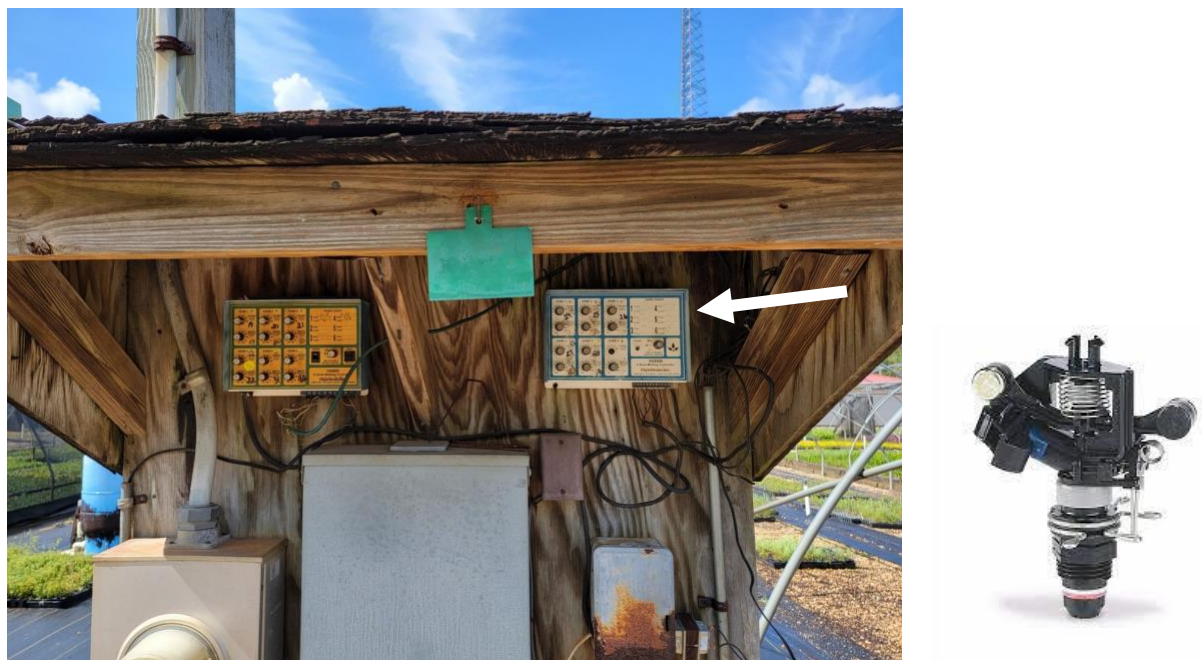
Figure 6. (left) Phytotronics 1626 Clock® controller (arrow) can mist up to 6-zones
