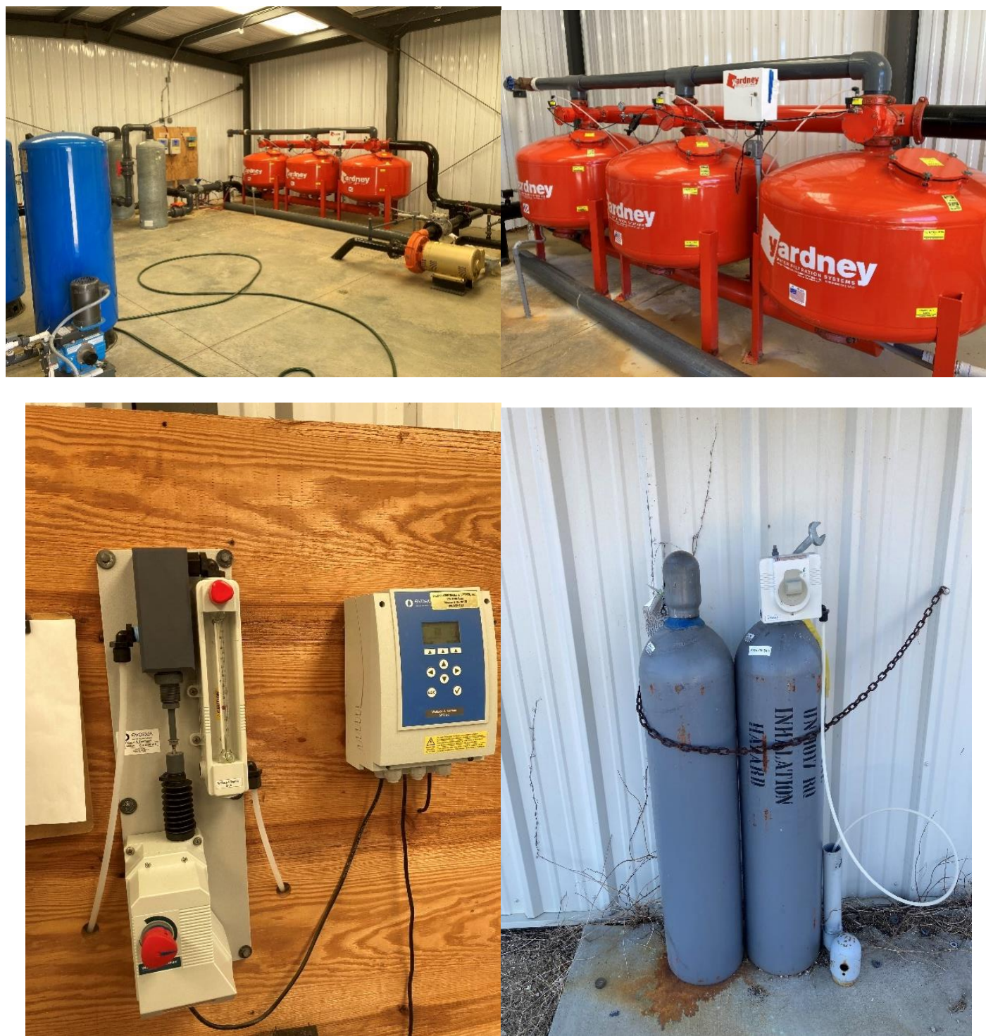
Figure 17. (top left) Interior view of pump house, (top right) a Yardney sand filtration system with automatic backflush, (bottom left) a Wallace and Tiernan® S10k gas feed chlorine metering system, and (bottom right) chlorine gas cylinders with regulator.
