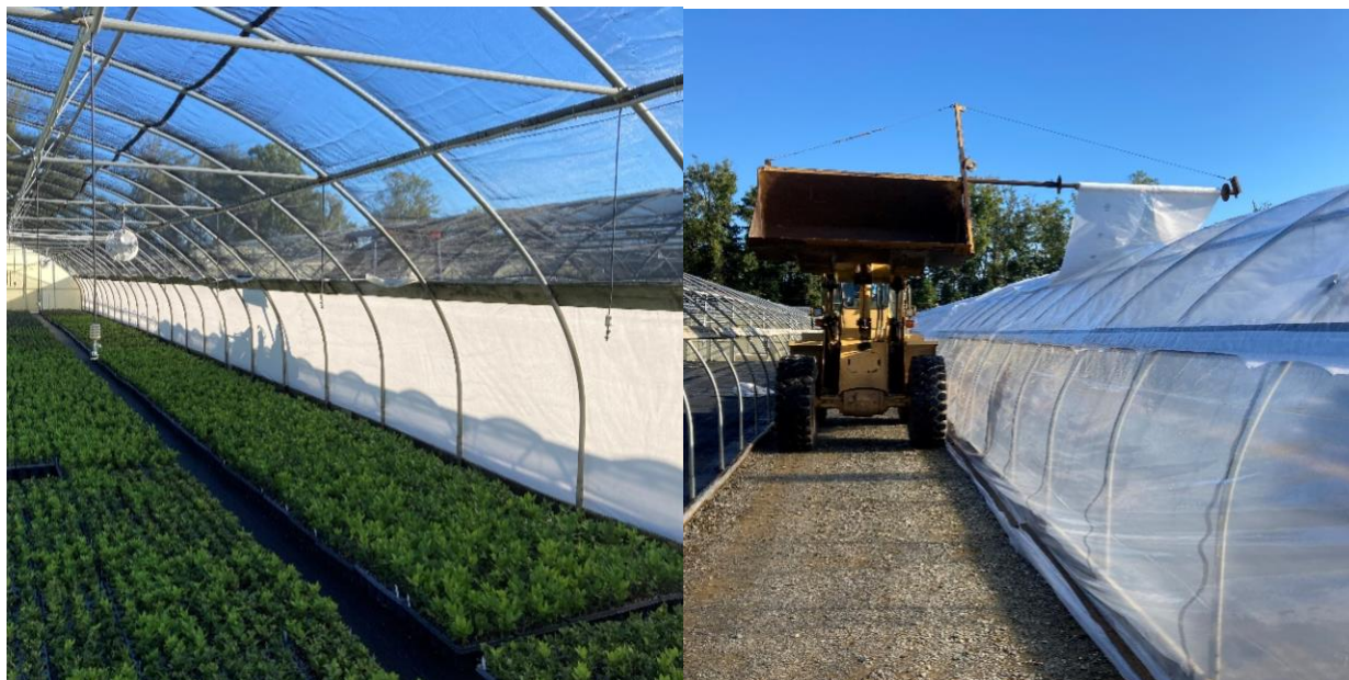
Figure 12. (left) A 9x44 m (30x145 ft) greenhouse covered with 50% shade cloth and 2 m (6-ft) plastic side curtains. (right) Applying a double layer of clear plastic to greenhouse using boom attachment.
