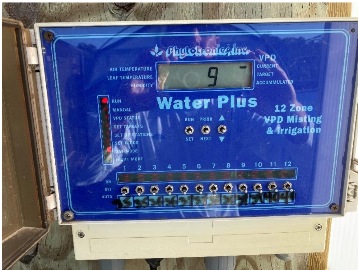
Figure 14. Phytotronics 12-zone vapor pressure deficit (VPD) controller.
