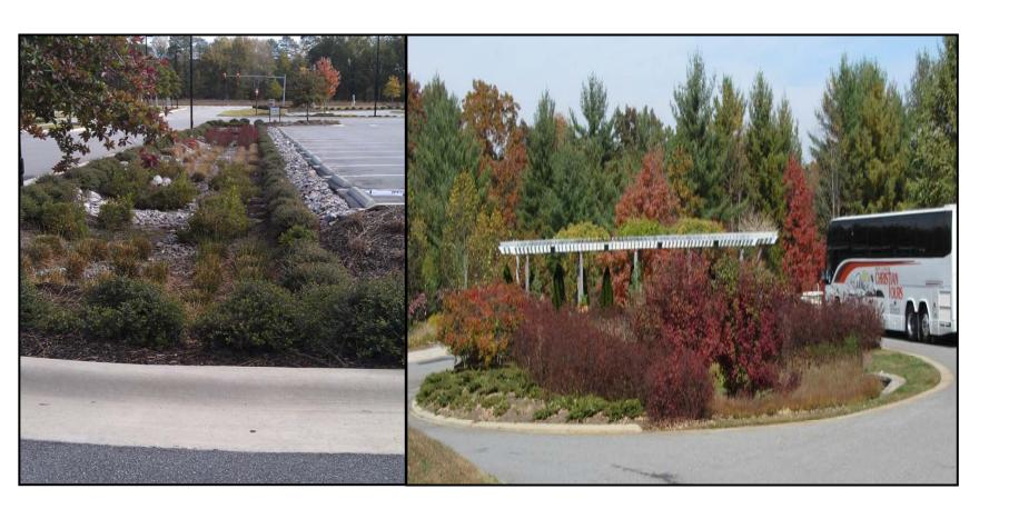
Fig. 1. Two rain gardens in North Carolina [Clayton, NC (left) and Ashville, NC (right)] with different designs, plantings and runoff collection from varying impervious surfaces.
